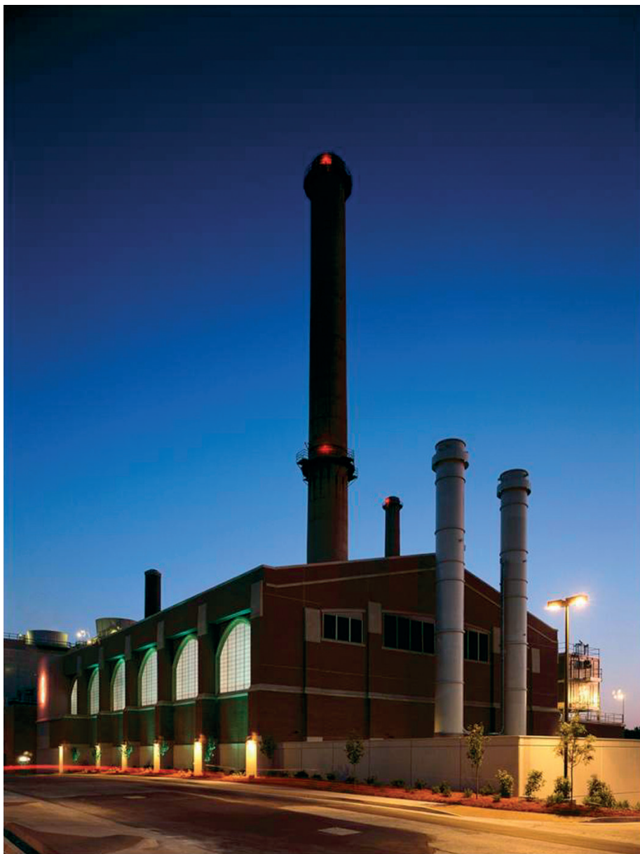
Figure 3: The University of Missouri, Columbia's award-winning power plant blends up to 10% of locally supplied woody biomass in its fuel mix.
