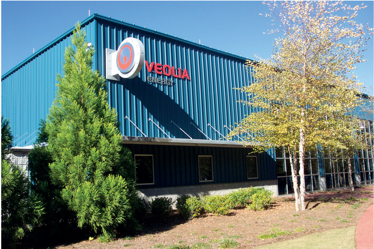
Figure 21: A central chilled water plant and district cooling network provide efficient air conditioning to the buildings in Atlantic Station, a model mixed-use development in Georgia
