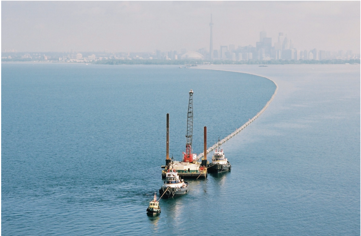
Figure 17: Enwave's Deep Lake Water Cooling uses the icy water of Lake Ontario to provide renewable cooling for the city of Toronto.
